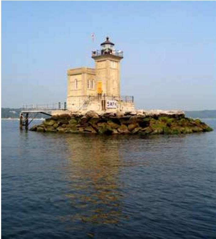
Harbor. In 1912, a new lighthouse was built to serve Huntington Harbor. The new structure was a unique lighthouse, in both design and construction. The Beaux Arts style makes the light look like a small castle. The reinforced concrete foundation and structure is unique to the area, as well. The foundation for the light was built nearby on land, then floated to the site and sunk.
